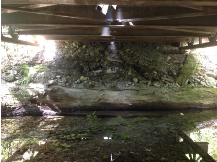
Right Bank Abutment when facing downstream
