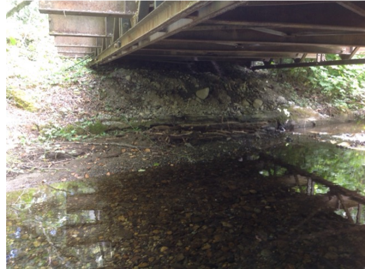
Left Bank Abutment when facing downstream
