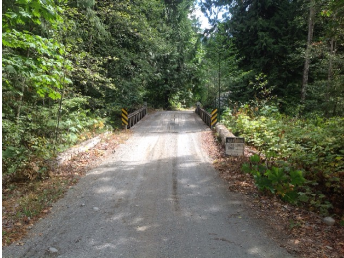
Approach from Right Bank when facing downstream
