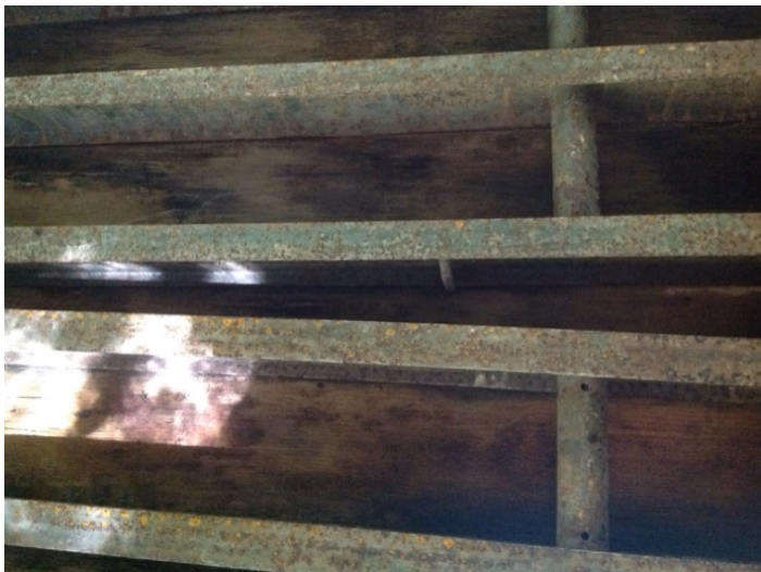
steel stringers are moving
